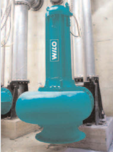
Dry sump installation
