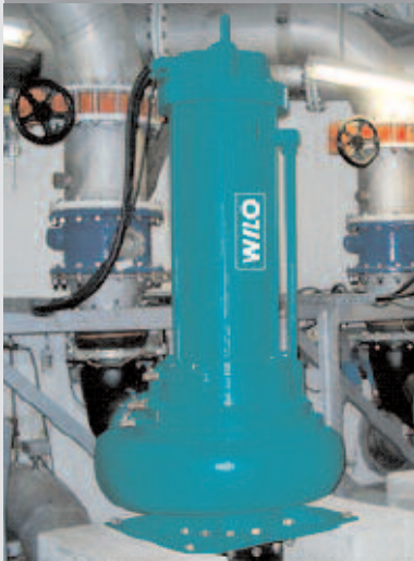
Dry sump installation
